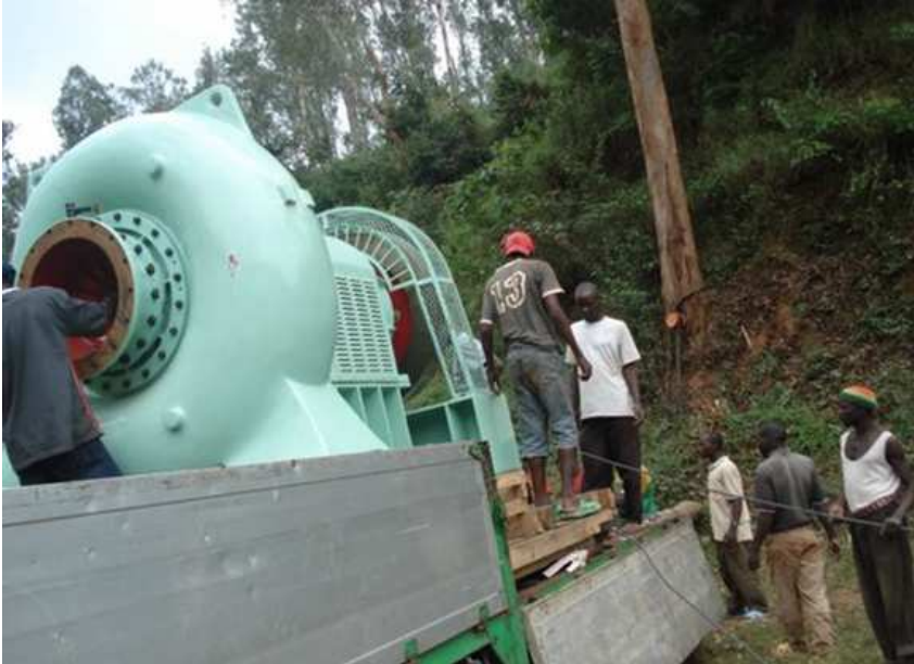
On-the-job training and capacity building on the project site.
