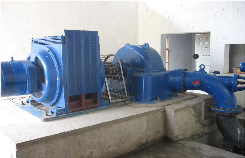
Mutobo Power house
