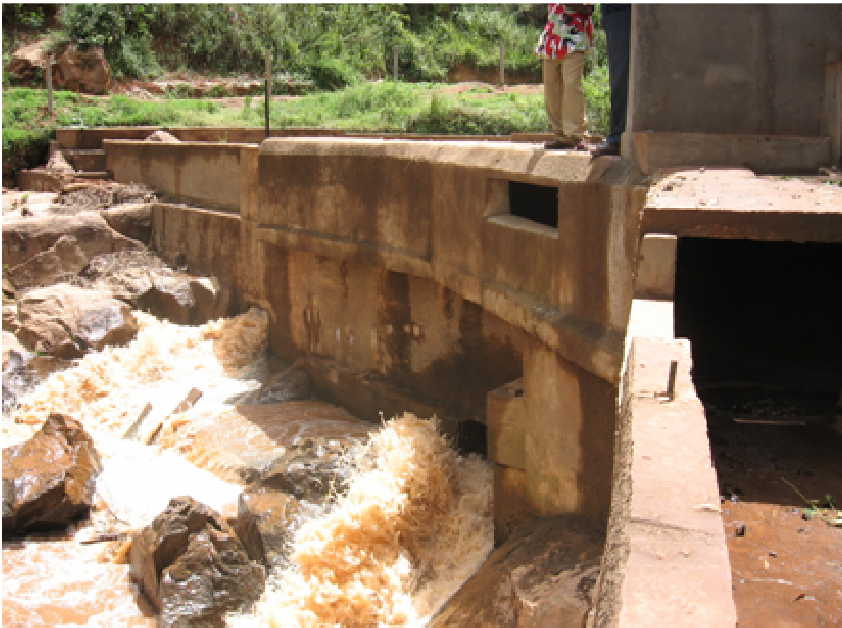
Special design arrangements to match the desilting needs of the river water
